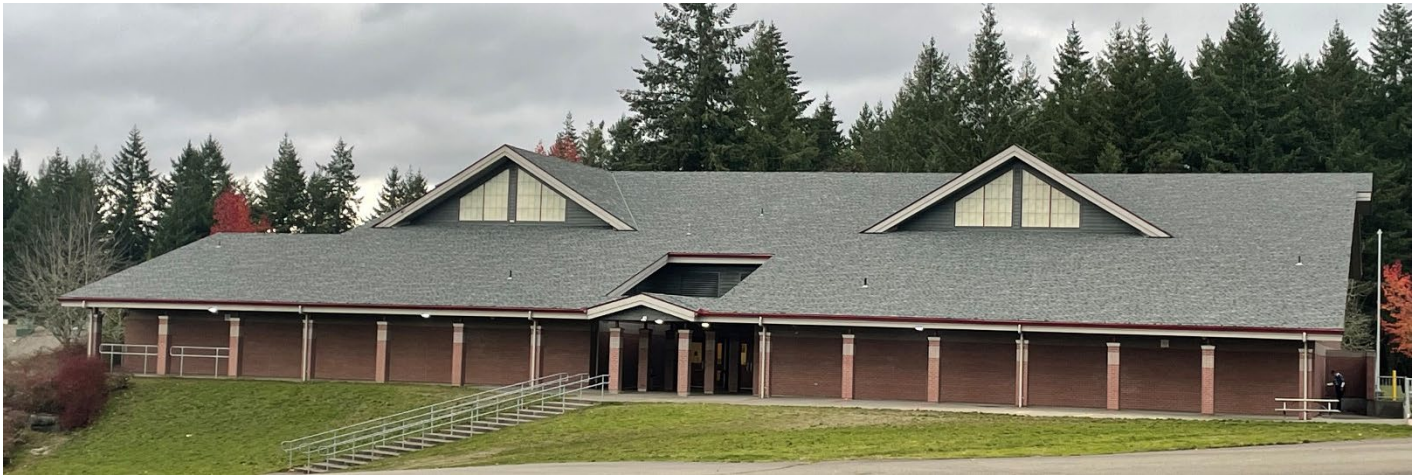
Below: The Gym building – photographer facing west.
